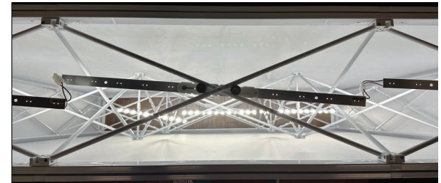
TOP VIEW OF LIGHT BAR INSTALLED AT TOP OF DISPLAY FRAMING
